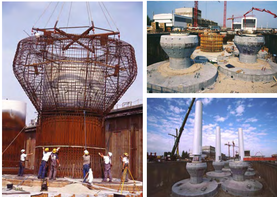
Middelgrunden Gravity Foundation Construction in Dry Dock Copenhagen, Denmark [35]
