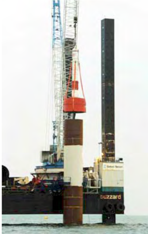
Monopile Driving at Horns Rev [32]
