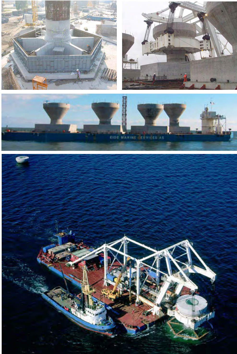
Gravity Foundations Under Construction and In Transit Nysted, Denmark Wind Farm [36, 37, 38]
