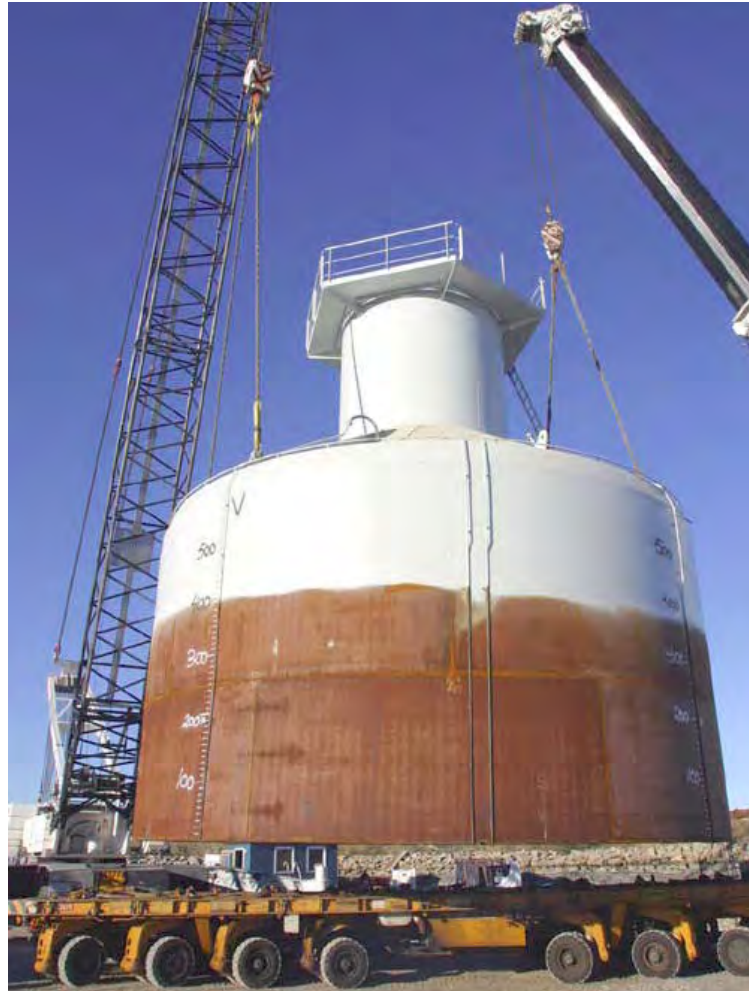
Prototype Suction Caisson – Frederikshavn, Denmark [43]
