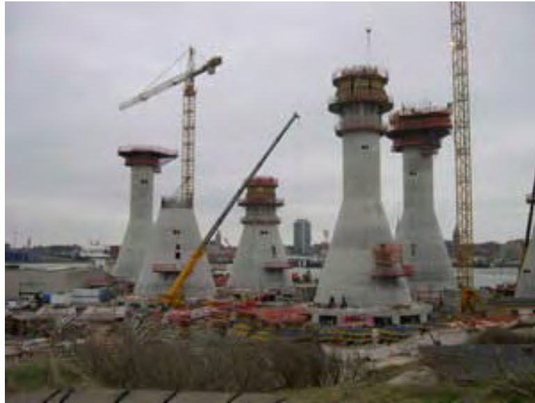
Gravity Foundations Under Construction Thornton Bank (Belgium) [39]
